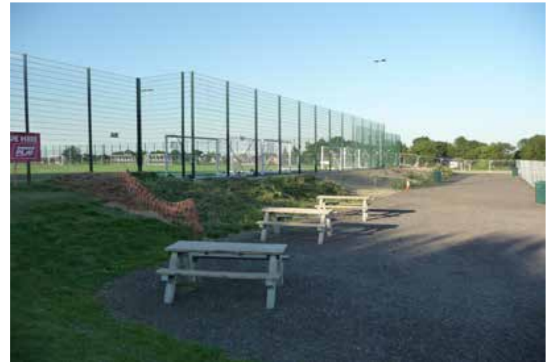
The new 3G artificial grass pitch, which is on raised ground.
